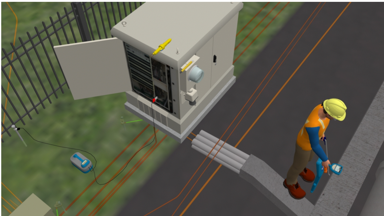
Direct Hook up to Digital Loop Carrier
